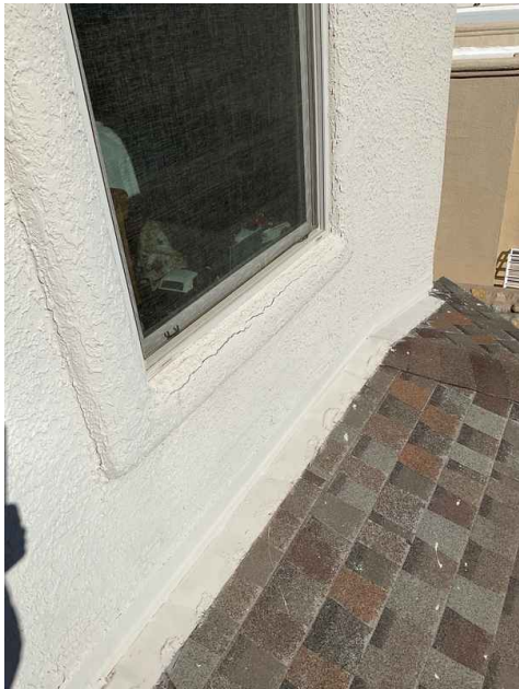
2nd Floor South Exterior Wall
