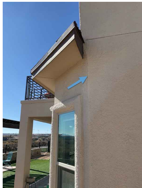
Southeast Exterior Wall
