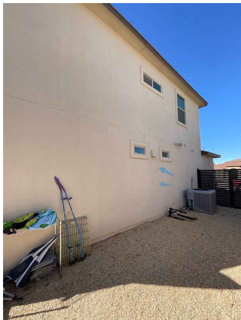
East Exterior Wall
