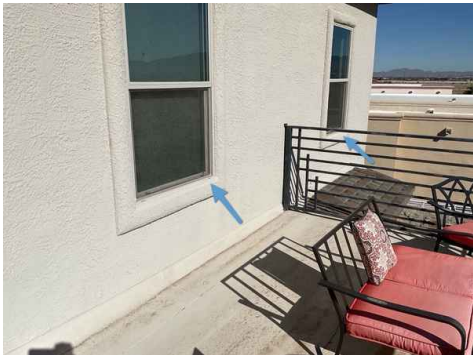
2nd Floor South Exterior Wall
