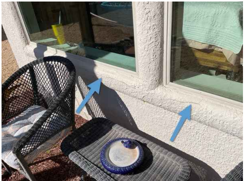
1st Floor South Exterior Wall
